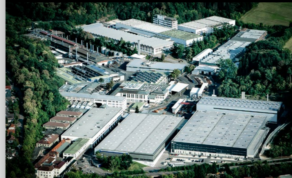
AERIAL VIEW OF MASCHINENFABRIK ALFING KESSLER GMBH
