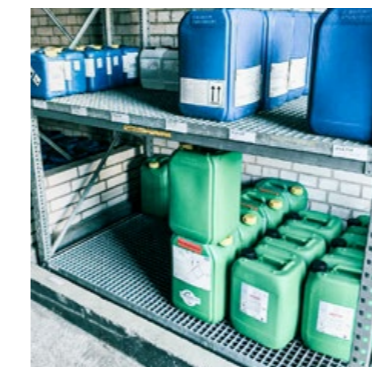
SECONDARY STORAGE OF HAZARDOUS SUBSTANCES
