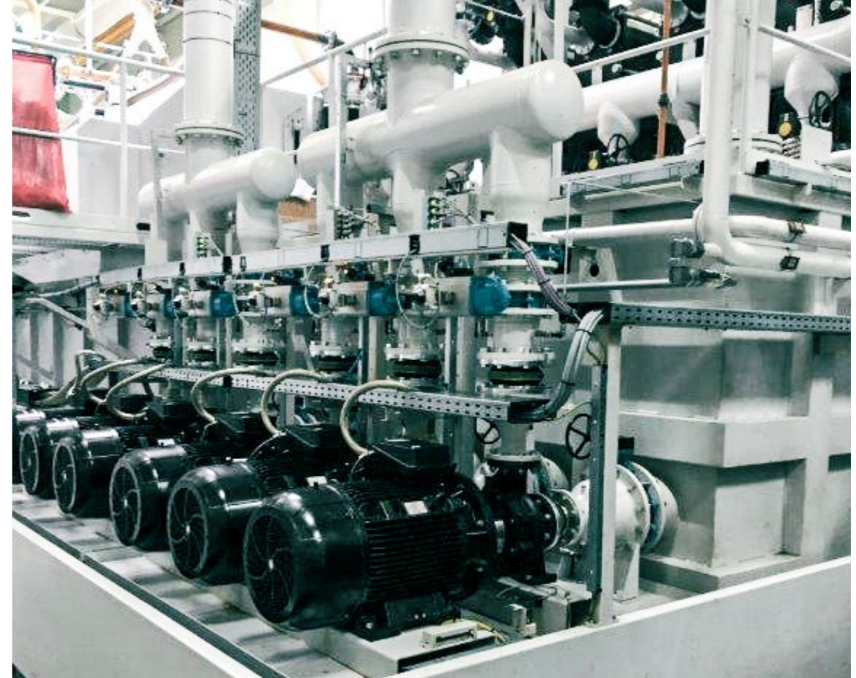
SECONDARY PROTECTION FOR COOLING LUBRICANT: CENTRAL UNITS
