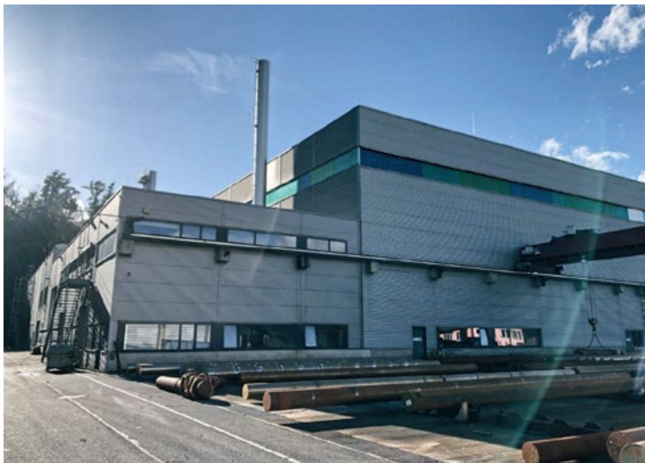
EXTERIOR OF FORGE SHOP LSUP
