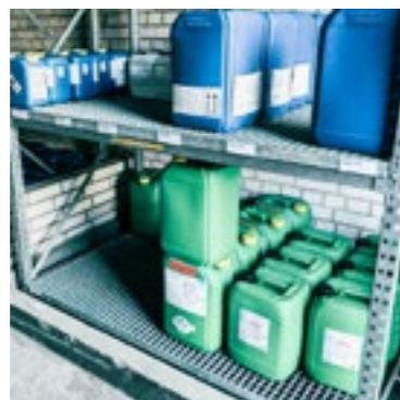
SECONDARY STORAGE OF HAZARDOUS SUBSTANCES
